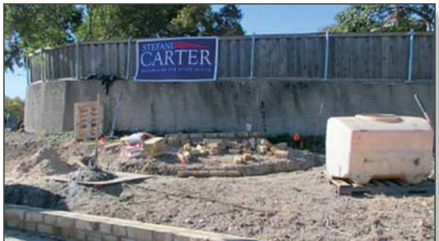
Nov. 6 – While voters go to the polls, a new retaining wall is constructed at the bottom of the slope and a footing is laid for the stone marker.
