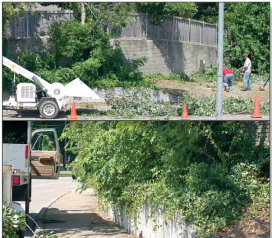
May – Dead trees, brush and debris are cleared from the work area. Design plans are submitted to the City for approval. Because the corner abuts an intersection, there are strict requirements regarding sight lines, set back, elevation and signage square footage area.
